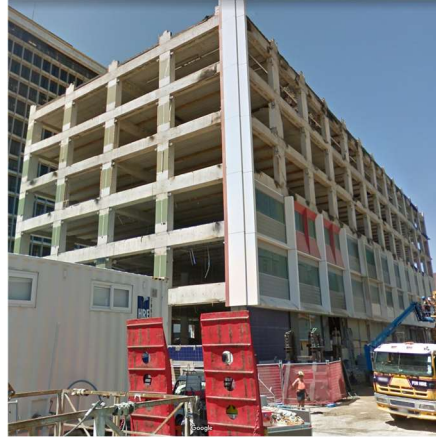
(b) Pre-2016 Kaikoura Earthquake, during demolition
