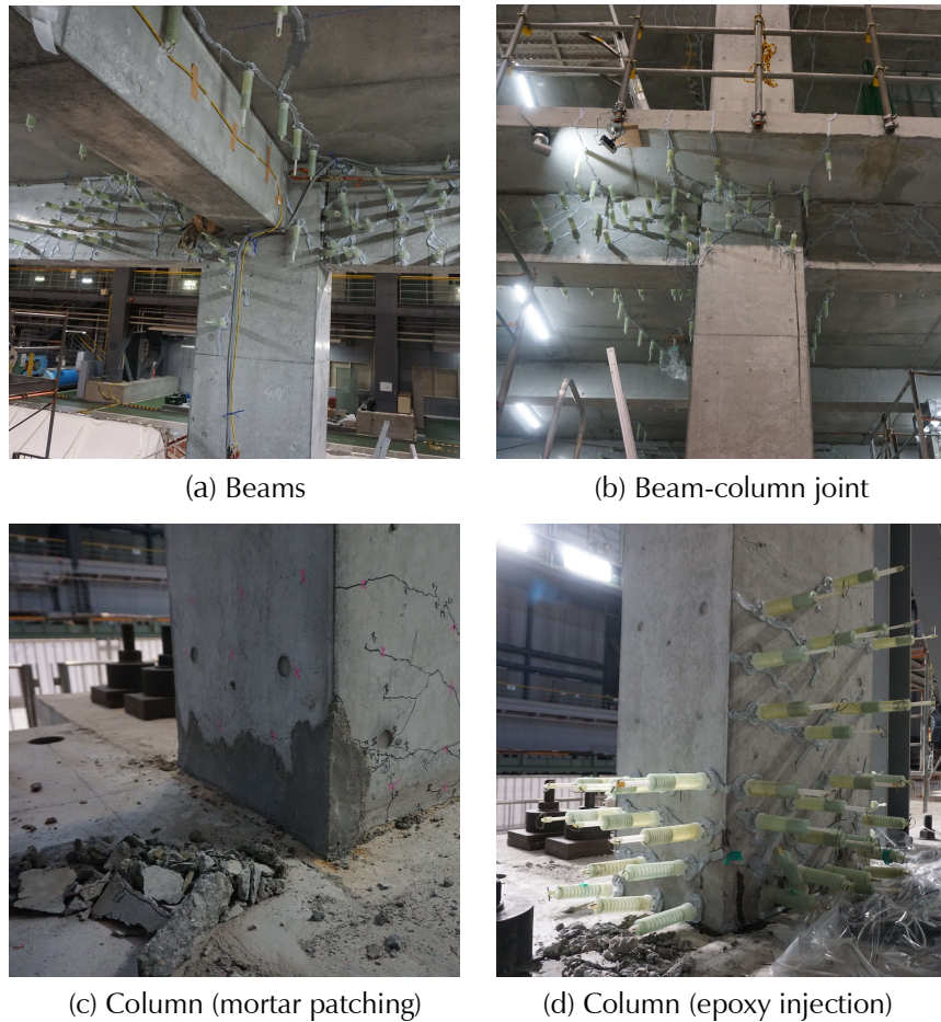
Figure 3-5 Epoxy injection and mortar patch.
